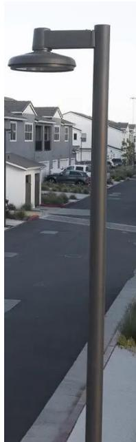
Description: Light pole assembly with 28' high pole and simple circular, disc style fixture
